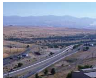
After: Magna Concentrator demolition
