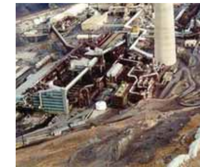
Before: Smelter footprint demolition
