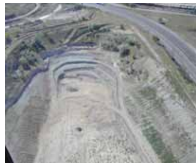
After: Sludge pond C excavation
