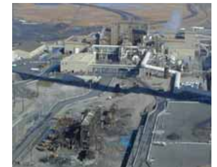
After: Smelter footprint demolition
