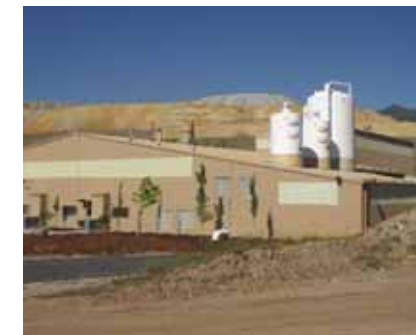
Bingham Canyon Water Treatment Plant
