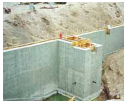
A typical east side water collection system cutoff wall during construction
