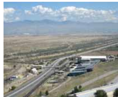
Before: Magna Concentrator demolition
