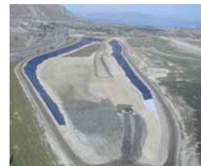
Arthur Stepback Repository during construction
