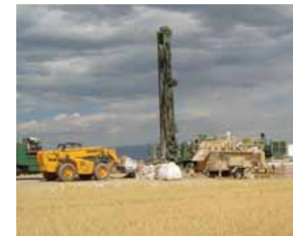
Groundwater extraction well during construction
