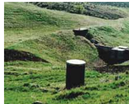
Completed cutoff wall
