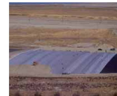
Capping of soil placed in Arthur Stepback Repository
