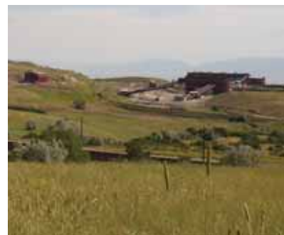
Before: Bonneville Crusher demolition
