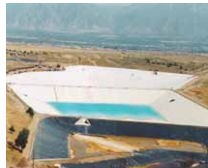
After: Large Bingham Reservoir reclamation
