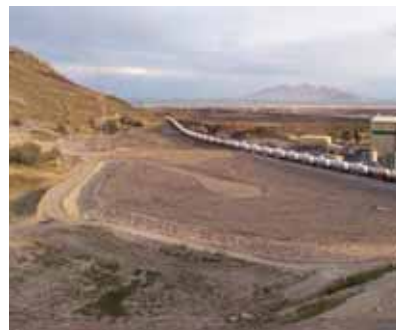
Refinery evaporation ponds cap in progress
