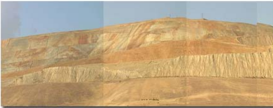
The Bluewater 1 dump in fall 2004 after being re-graded and contoured.
