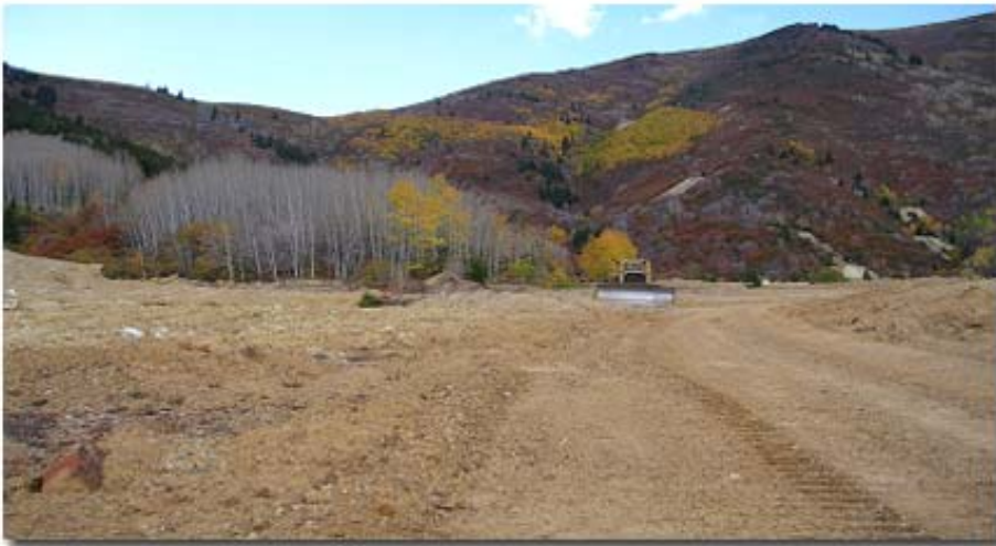
Highland Boy waste rock in Log Fork drainage looking west, showing ripped and contoured surface
