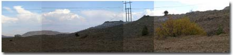
Highland Boy waste rock in Muddy Gulch looking north. The area has been contoured, ripped and volunteer vegetation preserved.
